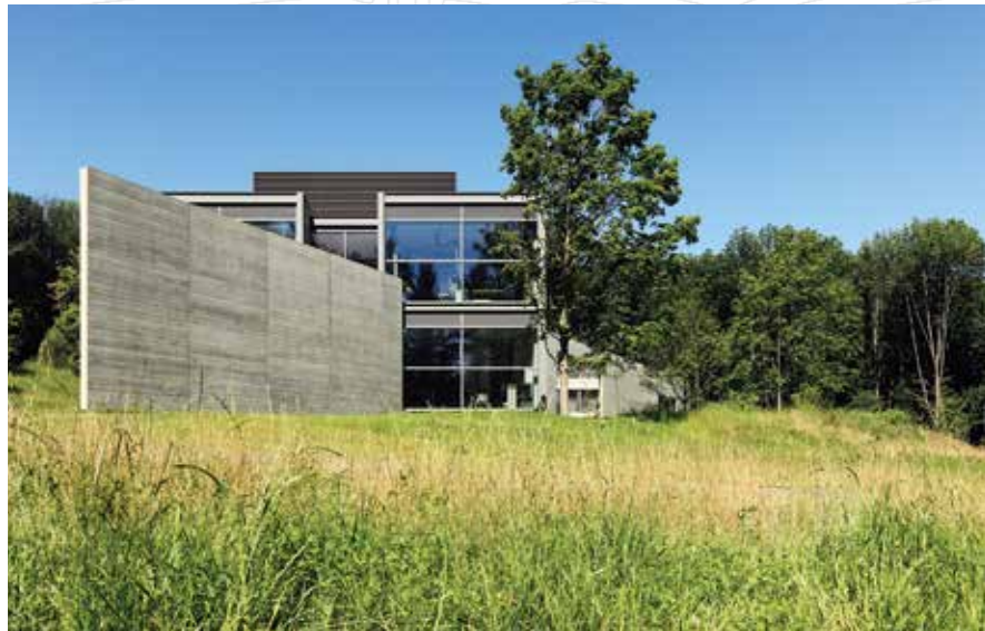
BELOW The lower terrace of grasses allows clear sight lines from the top-level conservation studios.
