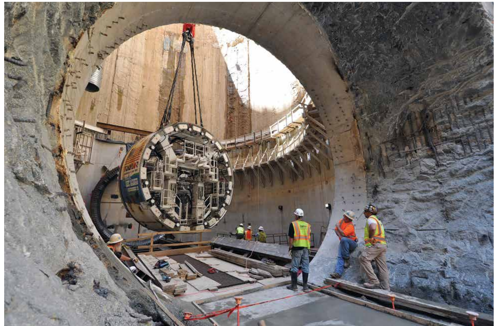
ABOVE DC Water's stable of charismatic boring machines now numbers four.
